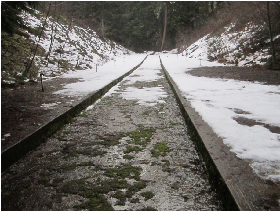
Concrete Spring Cap and High Flow Channel
