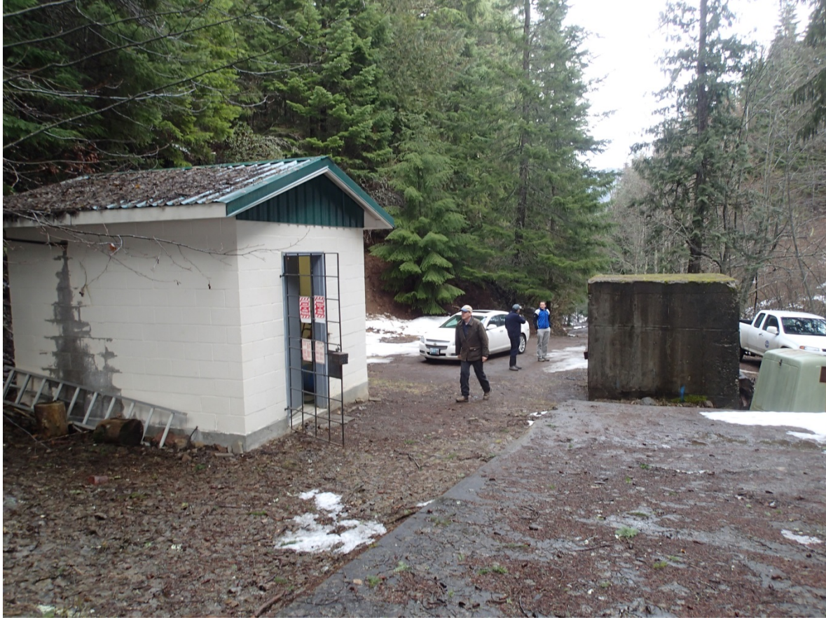
Disinfection Building (left); Intake Structure (middle right); Concrete Spring Cap (lower right)
